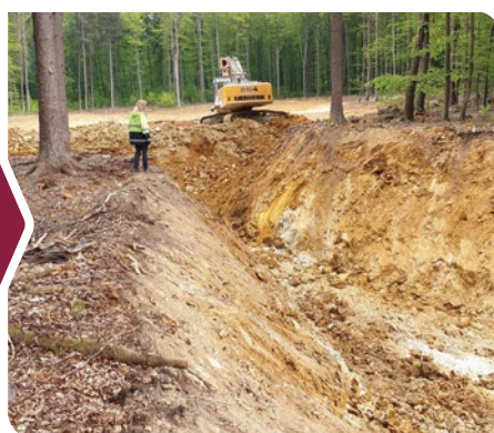
Aushub des Abraums Excavation of the 'overburden'
